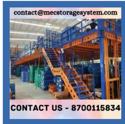
Mezzanine Storage Floor
